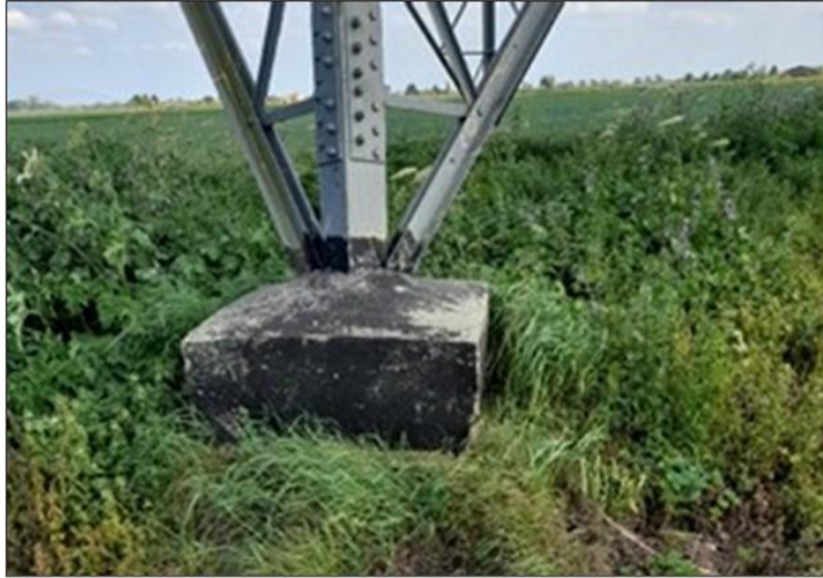
Plate 2.2 Typical pylon foundation base
